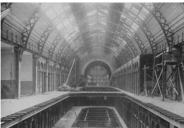
Figure 51 –Gallery shopfronts were brought forward and voids reduced in width
