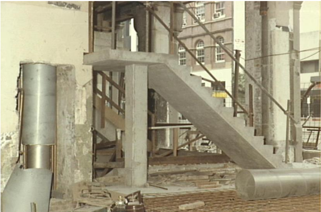
Figure 78 – Concrete stairs leading out to York Street
