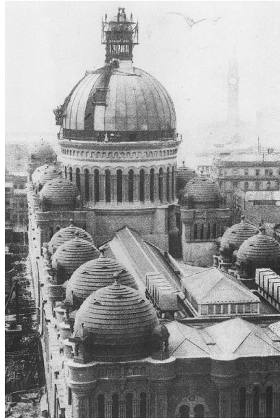
Figure 25 – The central dome nearing completion, c. 1898
