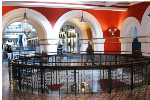
Figure 104 – The central drum and updated compliant balustrade
