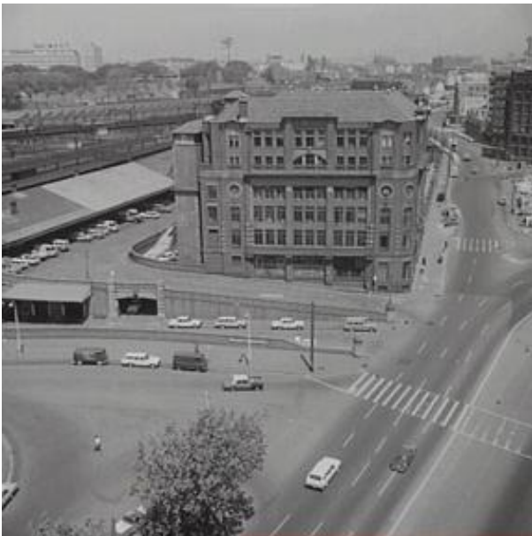
Figure 15 – Parcels Post Office at Railway Square (now operating as a hotel), 1967
