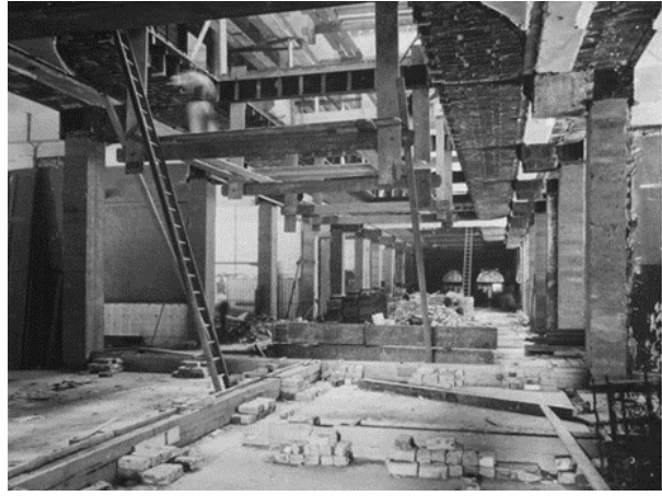
Figure 44 –Scaffolding and demolition materials, 1918 Source: City of Sydney Archives, NSCA CRS 51/2329
