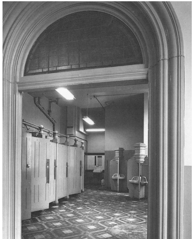
Figure 68 –Some of the men's bathrooms with their cast iron and porcelain urinals and partition posts were amongst the few internal areas to remain moderately intact
