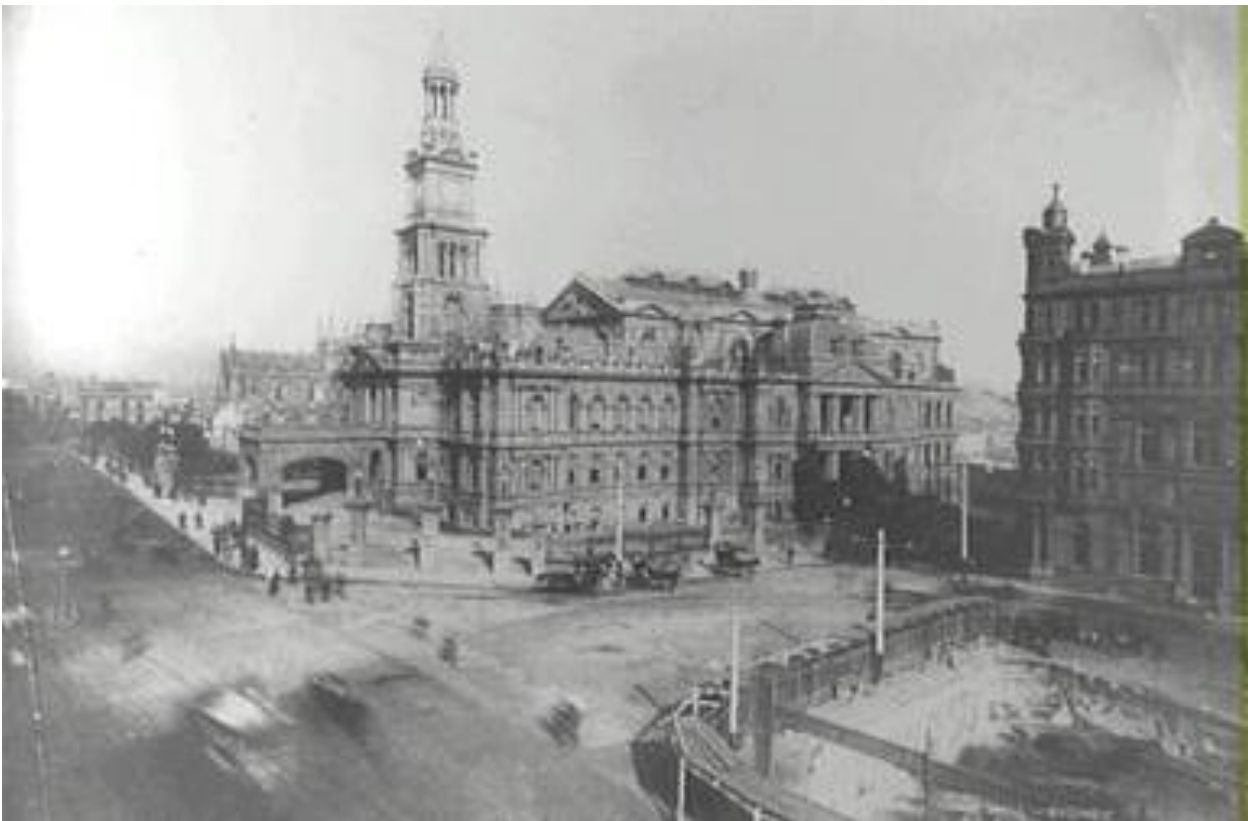
Figure 20 – Excavated site of the New City Markets (now known as the Queen Victoria Building)
