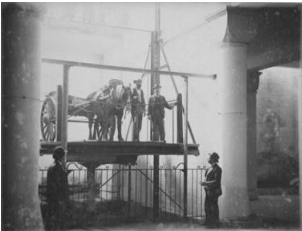
Figure 31 – One of the York Street lifts which serviced the basement livestock, fruit and vegetable market, 1898
