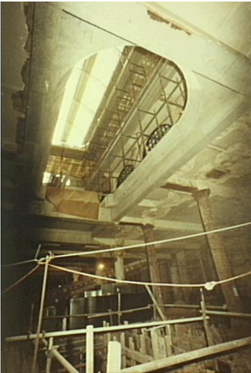
Figure 74 - Looking up from the ground floor through the newly recovered voids, 1985 Source: City of Sydney Archives, SRC11025
