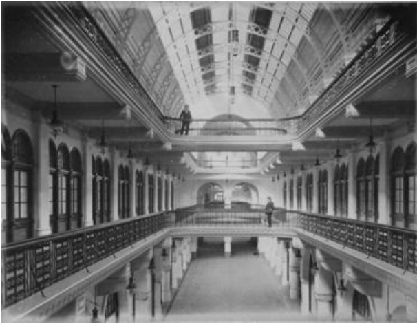
Figure 33 – View of ground floor, first and second floor gallery with details of joinery, railings and shopfronts, 1898
