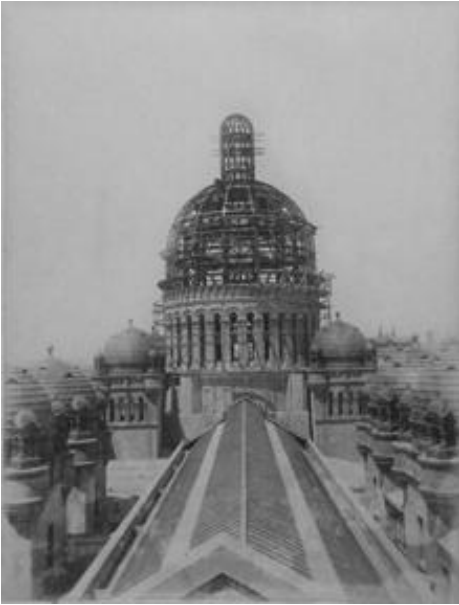
Figure 24 – View of the framing of the central dome, c. 1898
