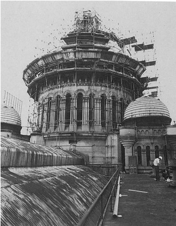
Figure 67 –The roof with corrugated iron still in place
