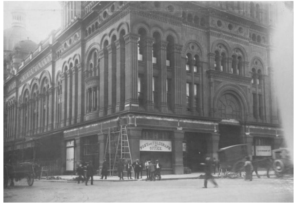
Figure 40 – Images of the 1918 alterations. Removal of the posted awning, 1918
