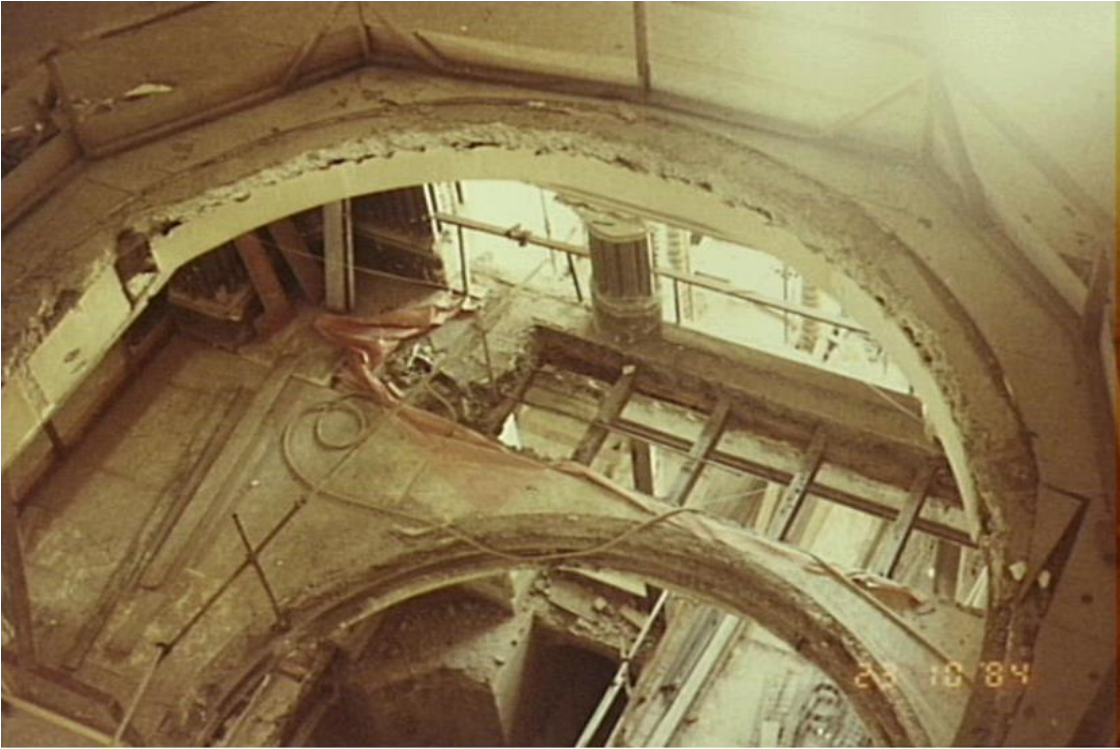
Figure 73 – Looking through the newly recovered central dome voids, 1984 Source: City of Sydney Archives, SRC10985
