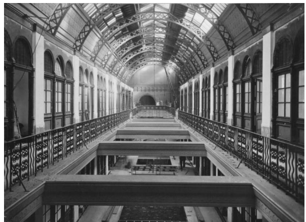
Figure 52 –Looking down into the reduced area of the south gallery, 1918
