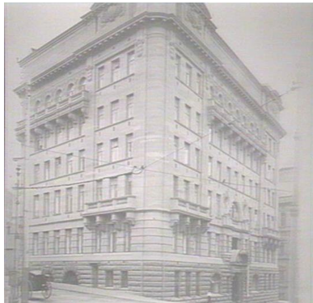
Figure 16 – Department of Education Building, 1915
