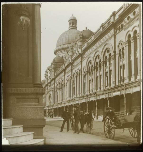
Figure 39 – Images of the 1918 alterations. View of the earlier posted awning that was removed, undated
