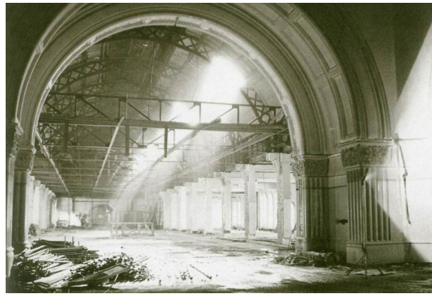
Figure 66 –The top floor at the commencement of works in 1984. The structure which supported the false ceiling under the barrel vault is evident and the concrete infills of the gallery voids had yet to be removed. Sheets of corrugated iron which replaced the original glass had been removed to allow light to be admitted
